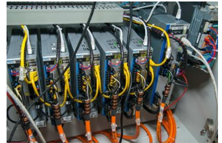
The AKD-C power supply unit (right) supplies the decentralized servo controllers. ME 2 also uses switch cabinet inverters from the AKD range to control additional drives outside of the rotary table.
