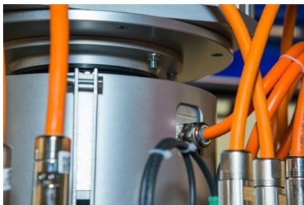
Inconspicuous but effective cable connection from the slip ring to the drive technology.
